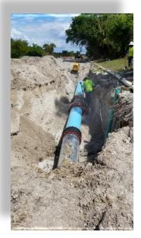
Force mains are pipelines that convey wastewater under pressure from one area to another
