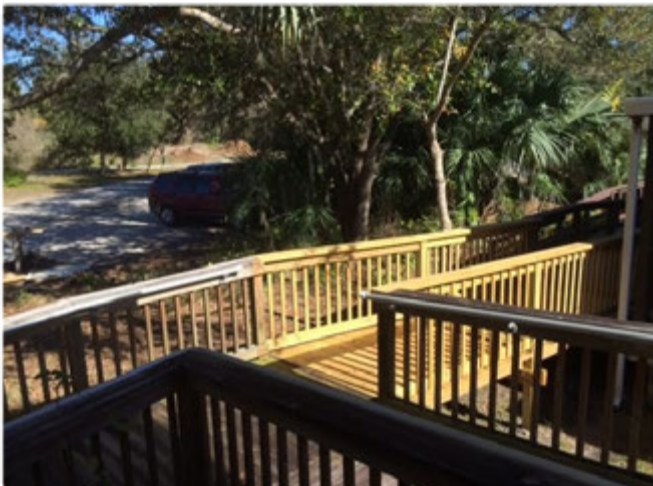
Above: New connector bridge
