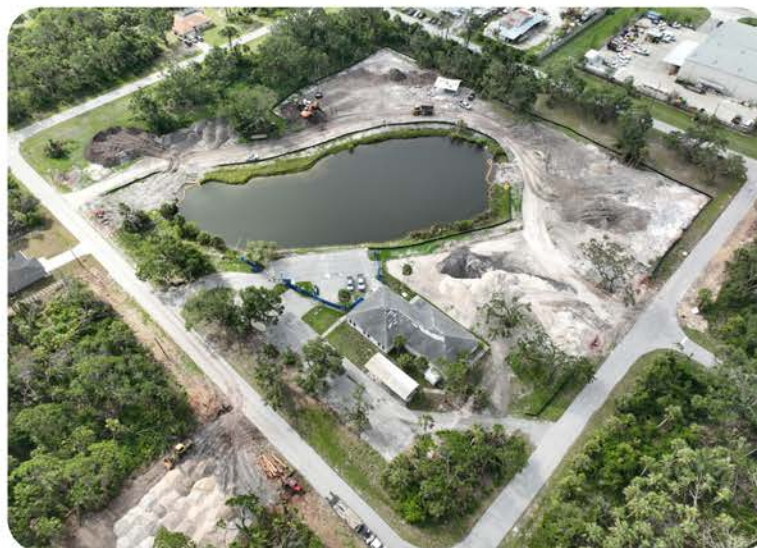
Photo: J.B. Yard under construction
