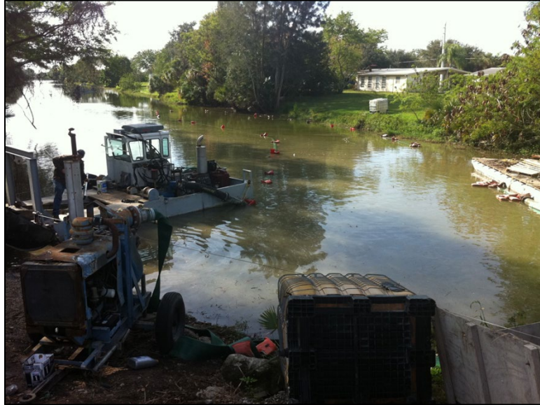
Figure 6. Photo of dredging operation in the Sunrise Waterway.
